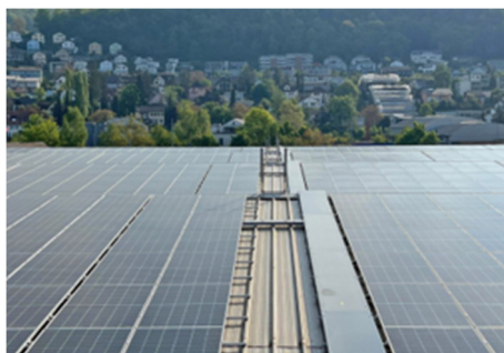
HIAG Solar plant in Brunegg
