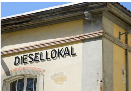
Former Windisch spinning mill
