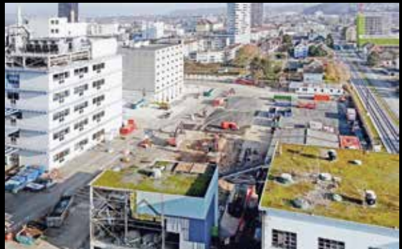
Chemicals successfully removed from the former Rohner site in Pratteln
