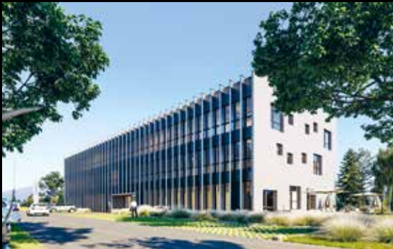
Construction begins on the Doka Switzerland office building in Niederhasli
